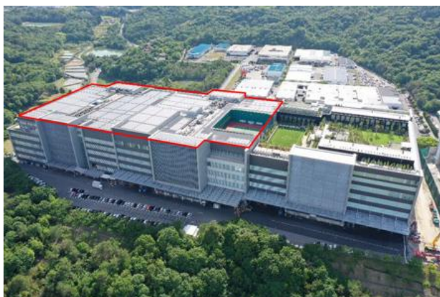
Solar power system at Kuwabata Plant
